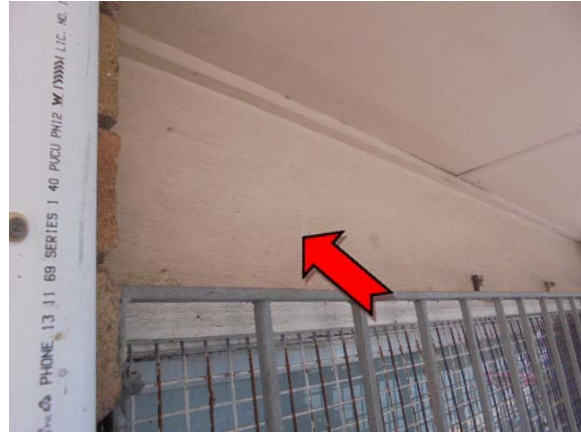
Photo 2. Exterior, northern windows, infill panels – asbestos-containing fibre cement sheeting.
